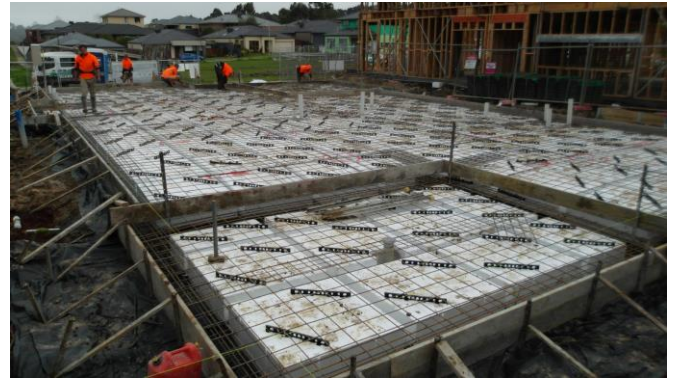
Typical Residential Foam Pod Slab construction using PodRail™
